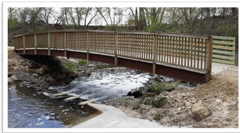
Figure 38: Upstream face of Bridge #1
