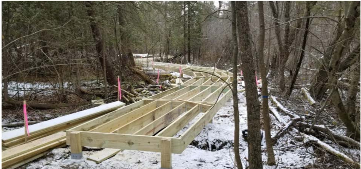
Figure 48: Example Bridge Pan style substructure. Pans are located at each of the posts on the snow
