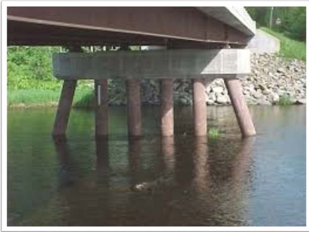
Figure 50: Example bridge bent pile pier substructure
