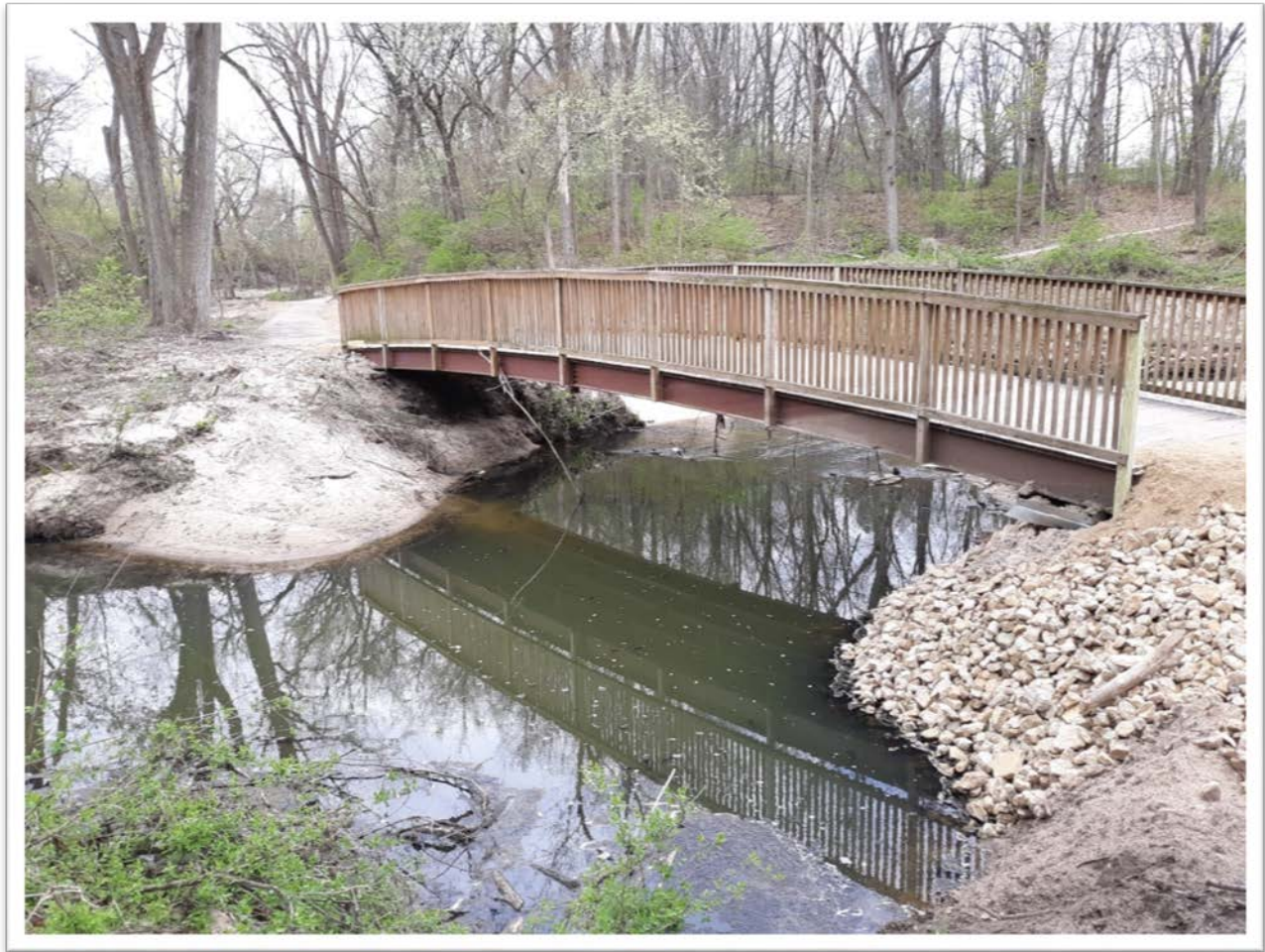
Figure 39: Upstream face of Bridge #2
