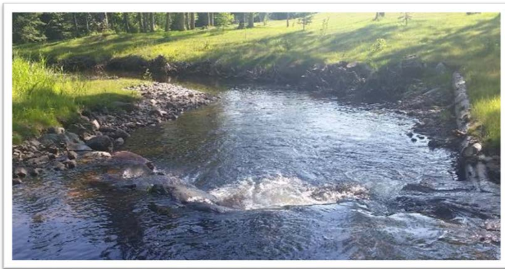
Figure 64: Example of rootwad log vane J-Hook combination installed by Cardno on the Knife River in 2016 near Two Harbors, MN
