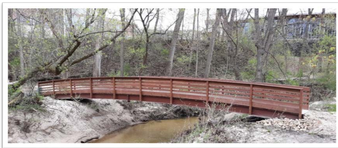
Figure 40: Upstream face of Bridge #3
