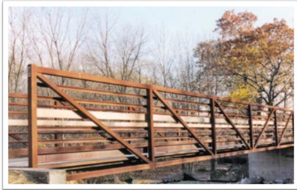
Figure 47: Example bridge railing style
