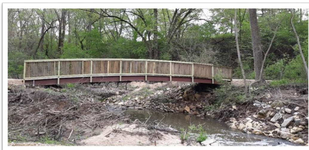
Figure 41: Upstream face of Bridge #4
