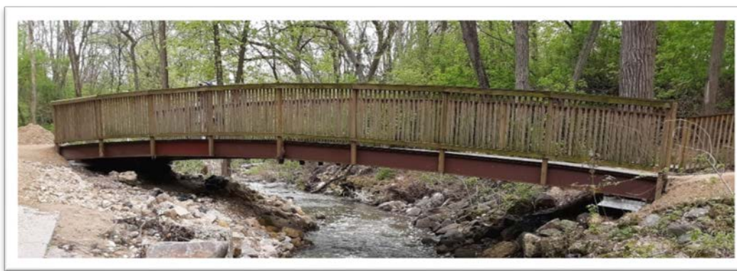
Figure 43: Upstream face of Bridge #6
