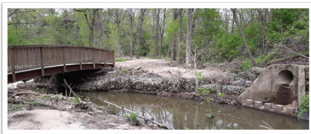
Figure 42: Upstream face of Bridge #5
