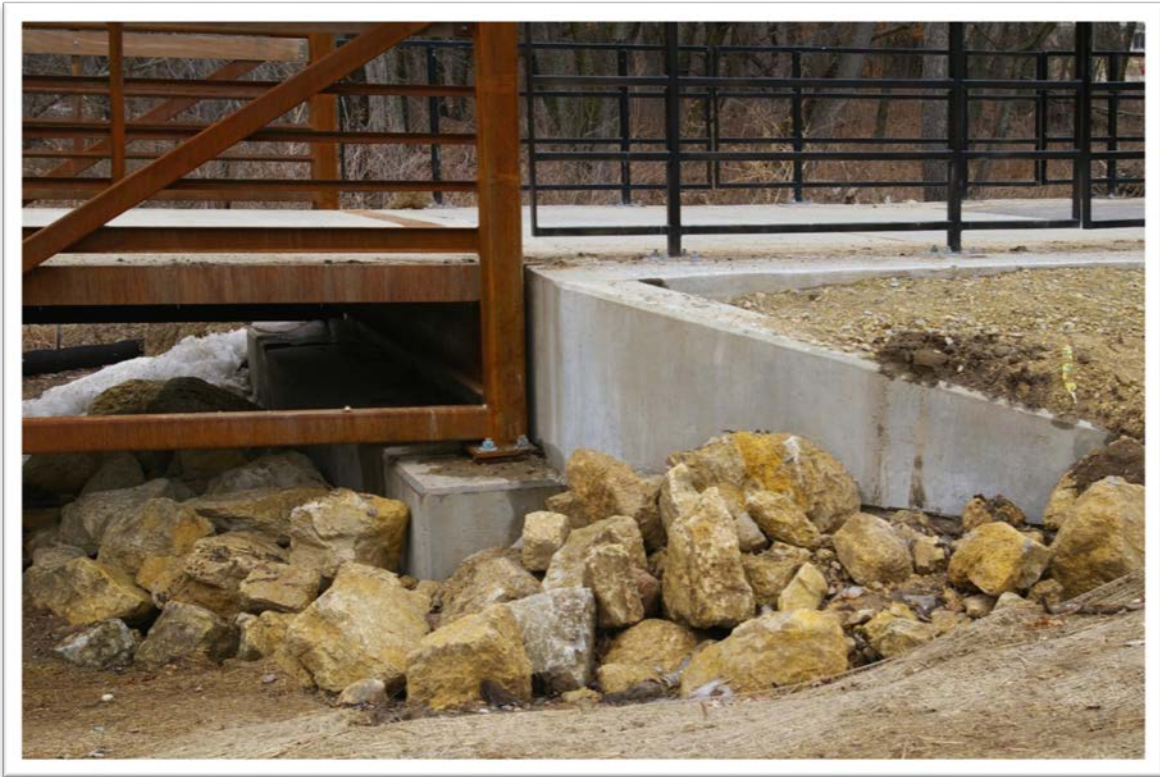
Figure 49: Example bridge concrete footing abutment substructure
