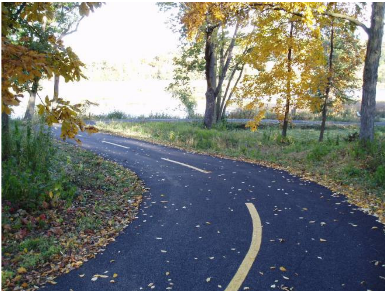
The Graber Pond Trail features porous asphalt that reduces surface water and is softer on runners' joints.
