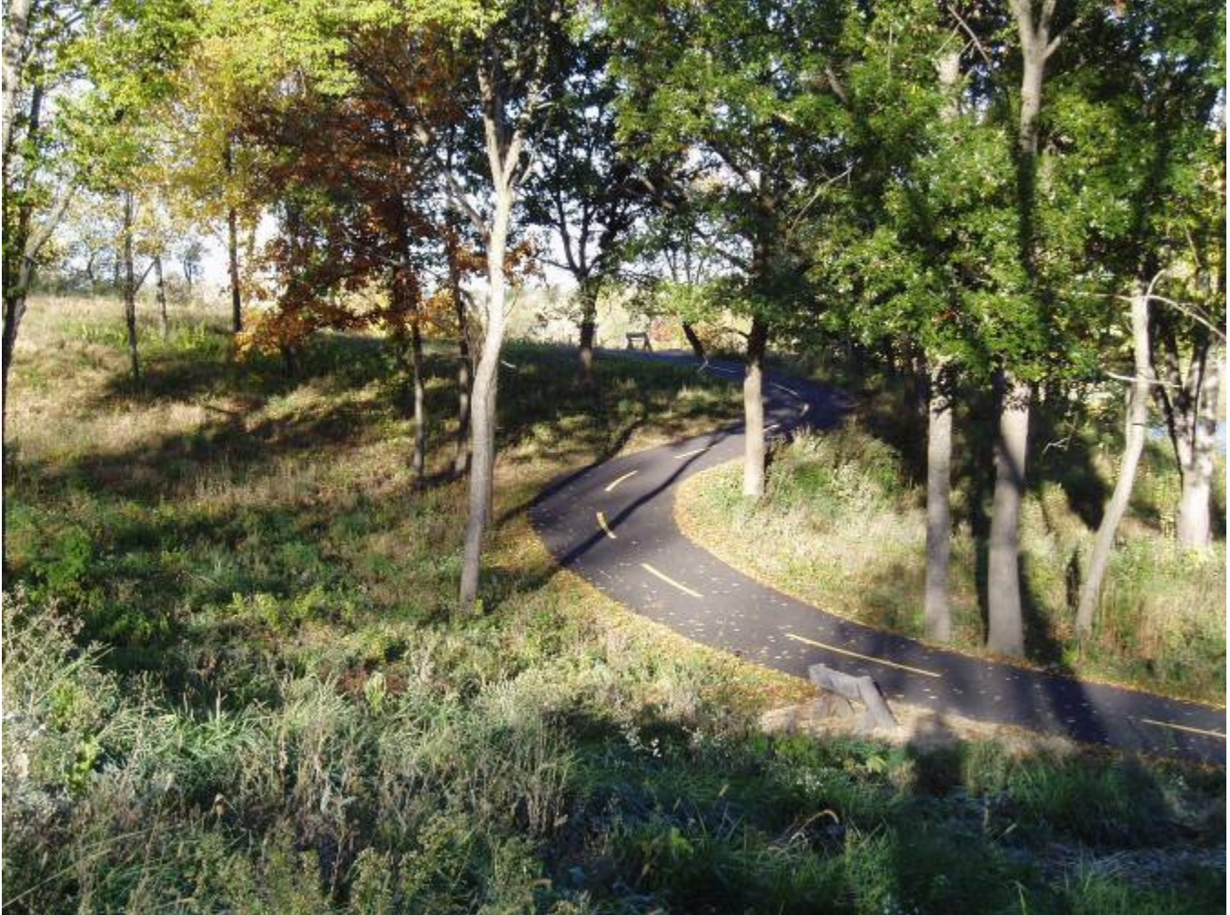
ADA maximum 5% longitudinal slopes required a sinuous alignment to navigate the rolling terrain on the south bank of Graber Pond.
